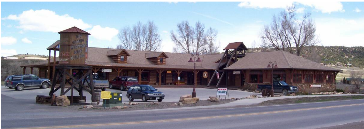
Southwest elevation, photo taken from Highway 62
