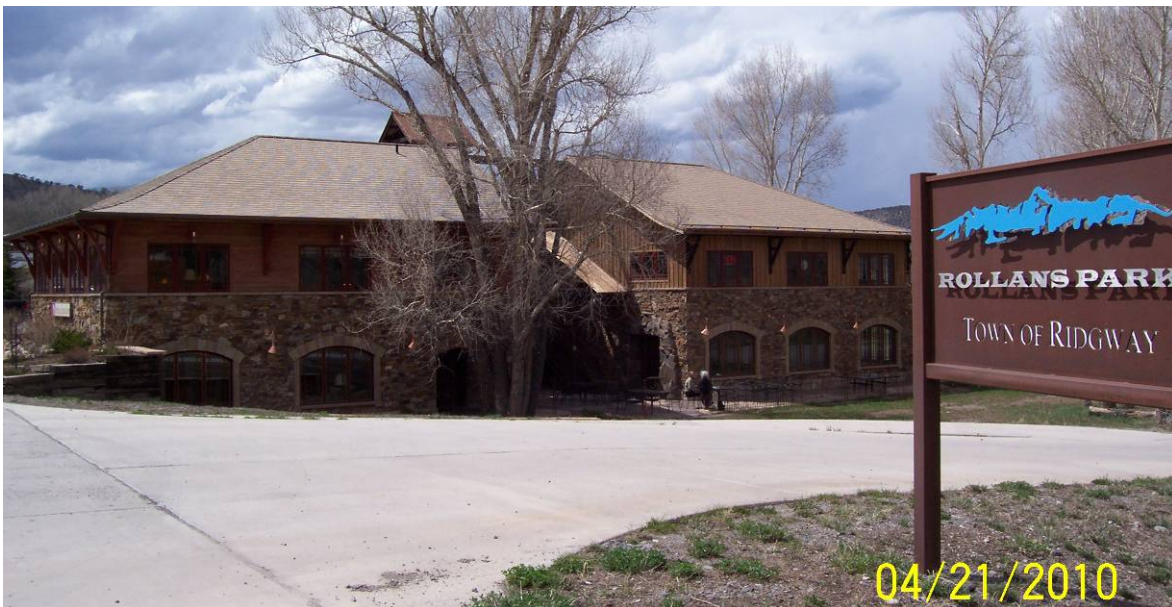
East elevation, photo taken from entry at Rollans Park/ Highway 62
